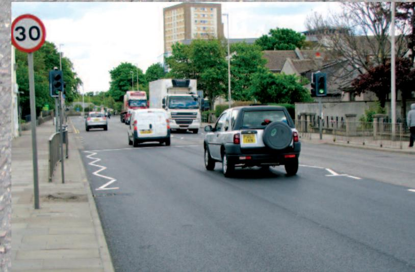
Leiths have developed a thin surface course system to cope with all aspects of surfacing from overlays to new pavement construction. The Rigagrip™ system consist of aggregate, filler and polymer modified bitumen. Mixtures are formulated to provide a dense durable mix with a surface texture to provide high levels of skid resistance.
