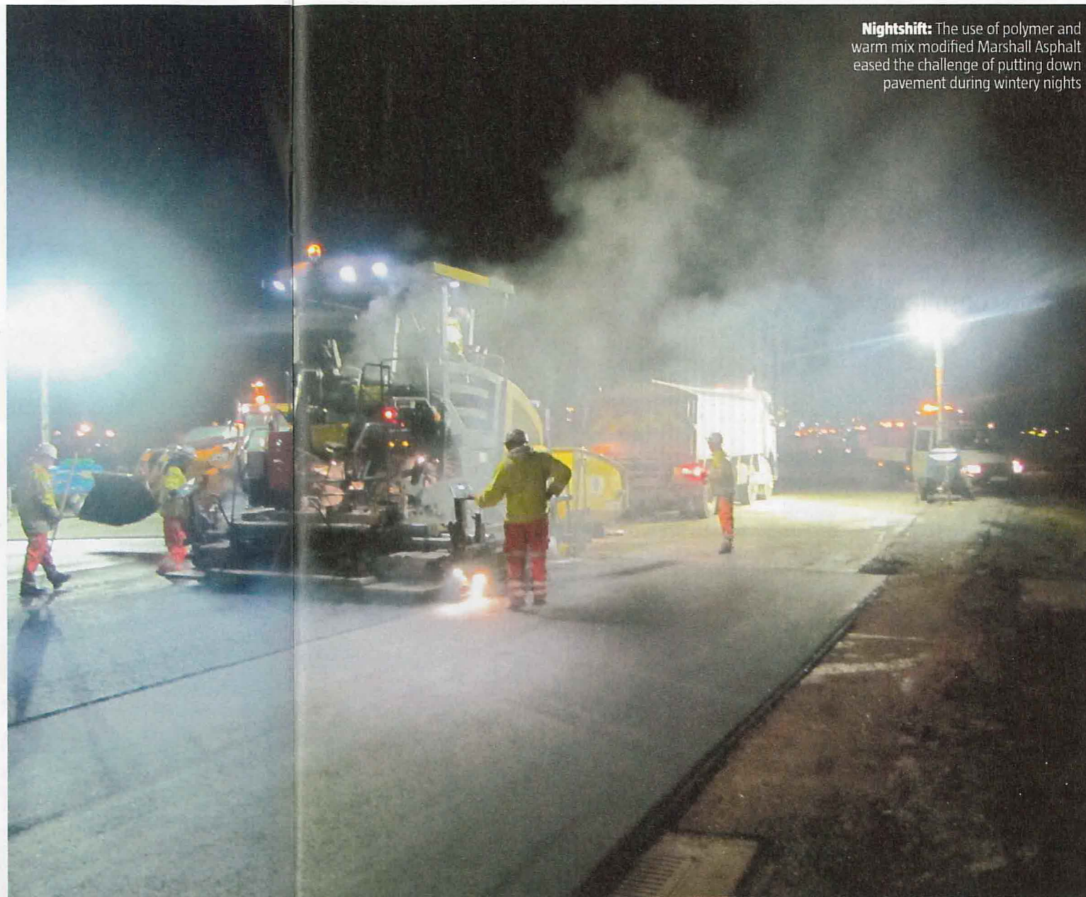
Taxiway strengthening: The initial warm mix layer is placed atop existing concrete
