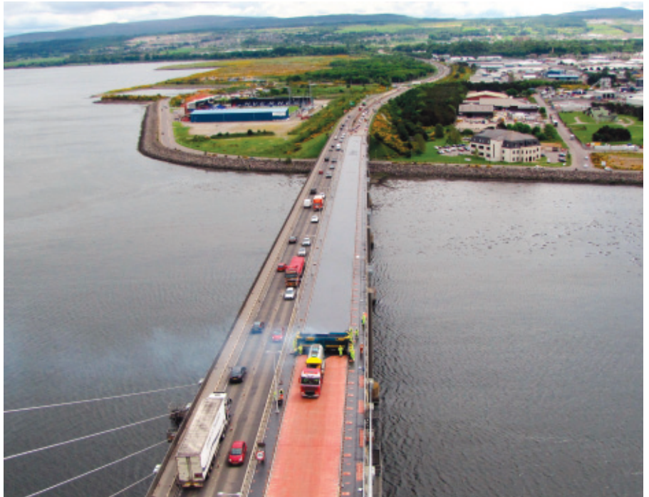
Surfacing going down on Kessock Bridge, which spans the Beaully Firth on the A9 north of Inverness
