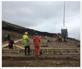
The helicopter delivering the Fibre Mix via Bucket connected to a linch. The Fibre Mix is positioned in place and poured. The Fibre Mix contained 3kg/m3 of macro synthetic fibre Durus EasyFinish.
