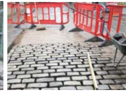
Reconstruction - in progress
