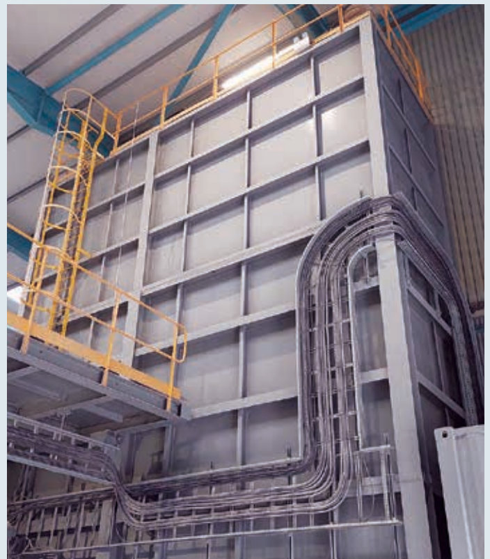
Aggregate hopper complete and installed at Highland Lime.
