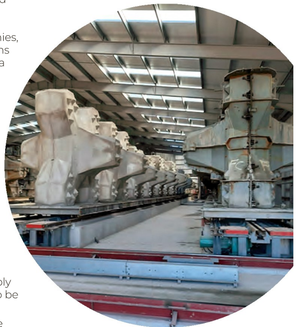
ABOVE: Casting of the accropode units.
