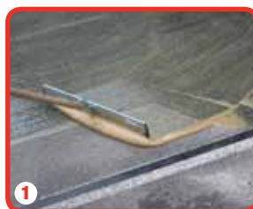
1 Area is cleared of debris and marked with tape before resin and hardener mix is spread over it
