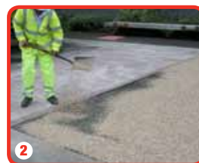
2 Appropriate aggregate is broadcast over the resin mix
