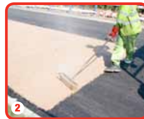
2 High friction surface is spread evenly and levelled
