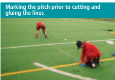
Marking the pitch prior to cutting and gluing the lines
