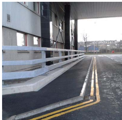
Pictures show the completed frontage to the new office development and also the steel reinforcement required for the vehicle barrier system designed to stop an articulated lorry from crashing into the building.
