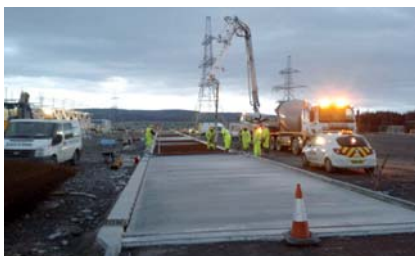
Civils squad pouring a section of concrete road
